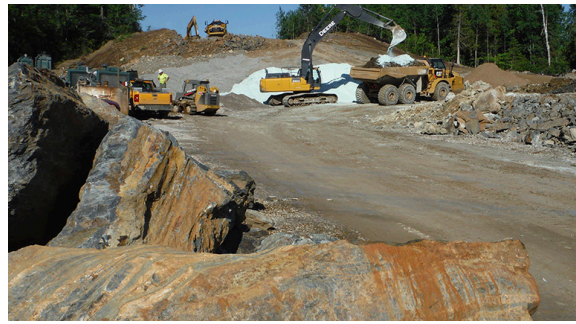
For MnDOT's highway construction project, Barr helped implement an ARD mitigation plan that tested pyrite-laden rock for sulfur, and if needed, mixed it with lime and placed it in fill areas covered with geomembranes to neutralize the potential for acid leachate.
